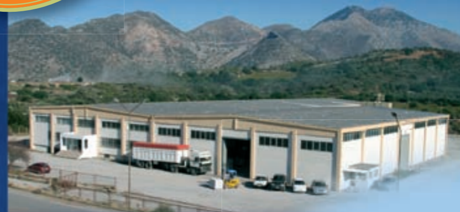
Industrial Area 4.500m 2
