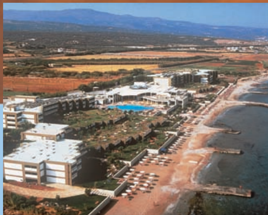
PROJECT: Full reconstruction of plastering in El Greco (Grecotel) hotel • Choice: A3
